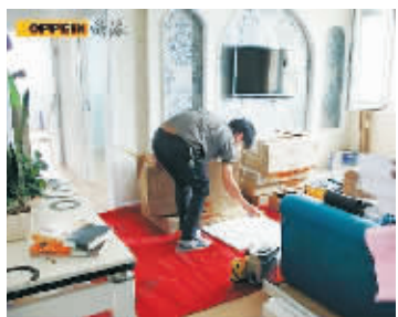
师傅在安装地柜
